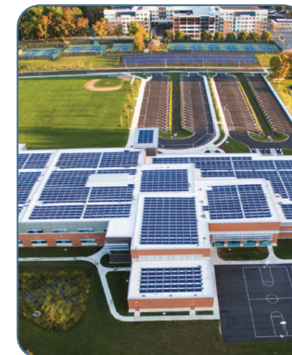
WILDE LAKE MIDDLE SCHOOL | COLUMBIA, MD PHOTO CREDIT: JAMES POSEY ASSOCIATES
